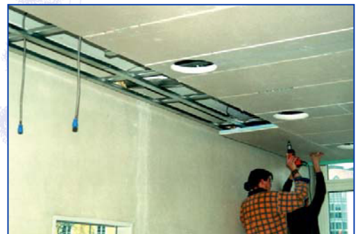
BEKA cooling ceiling with dry-built prefabricated elements
