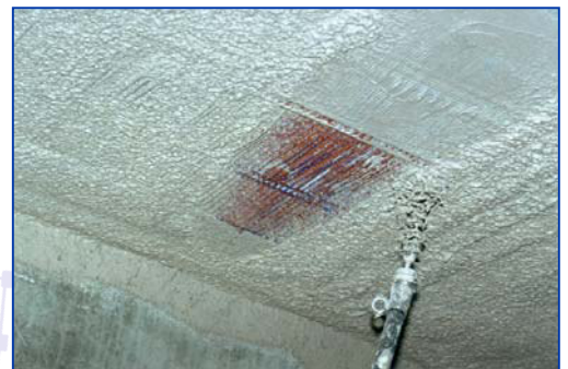
BEKA cooling ceiling as plaster ceiling
