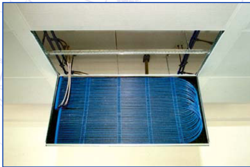
BEKA cooling ceiling as metal cassette ceiling
