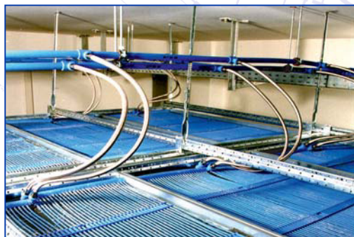
BEKA supply lines with quick-action couplings
