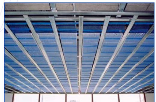
BEKA cooling ceiling as dry-built-ceiling
