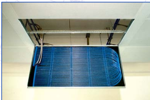
BEKA cooling ceiling as metal cassette ceiling
