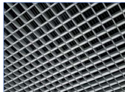
Nearly invisible: uncolored capillary tube mats unite with the open ceiling construction
