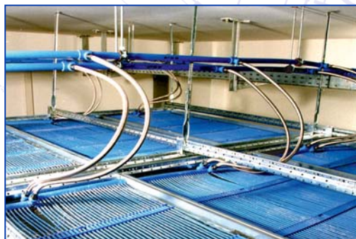
BEKA supply lines with quick-action couplings
