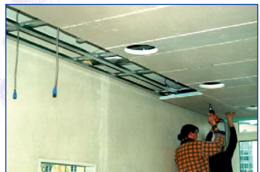
BEKA cooling ceiling with dry-built prefabricated elements
